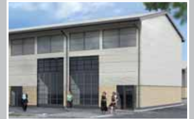
Rear elevation showing full height access door
